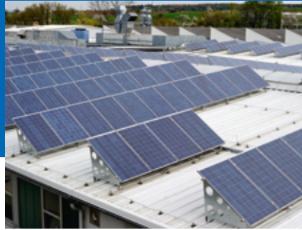
250 KW – Photovoltaikanlage
